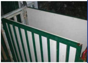
Plastic lining in stun box area to insulate electrical current.
